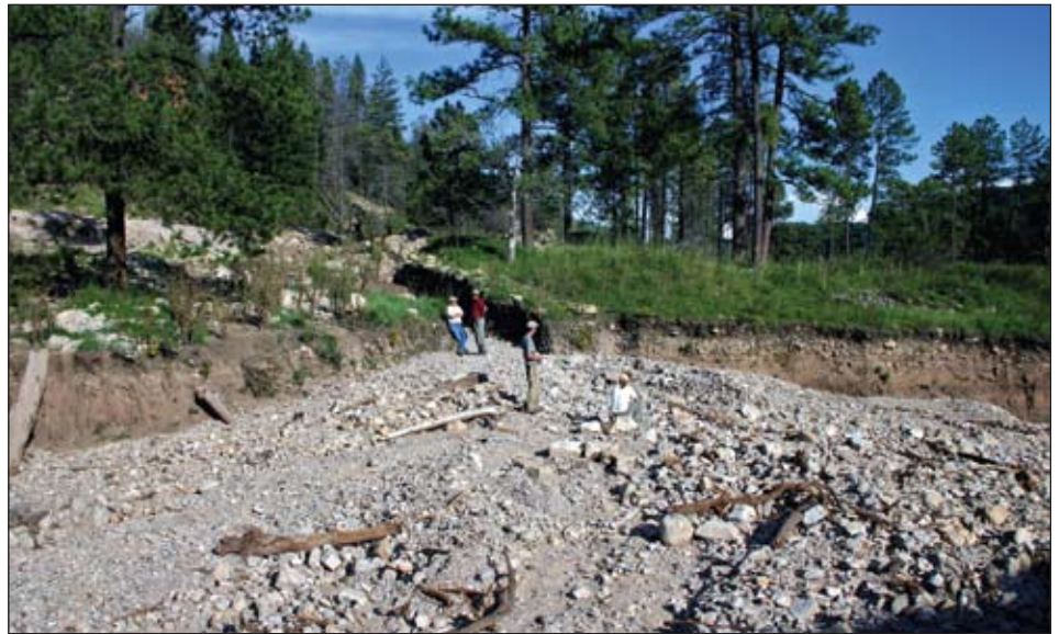
FIGURE 1—Deposits of a debris flow from a tributary basin of lower Cox Canyon in the Sacramento Mountains. The tributary basin was severely burned in the 2002 Peñasco fire. Debris-flow deposits partially filled and dammed the main valley arroyo at this location (the arroyo wall is visible across the center of the photo). The surface deposits lack mud because of reworking by later flood flows.
