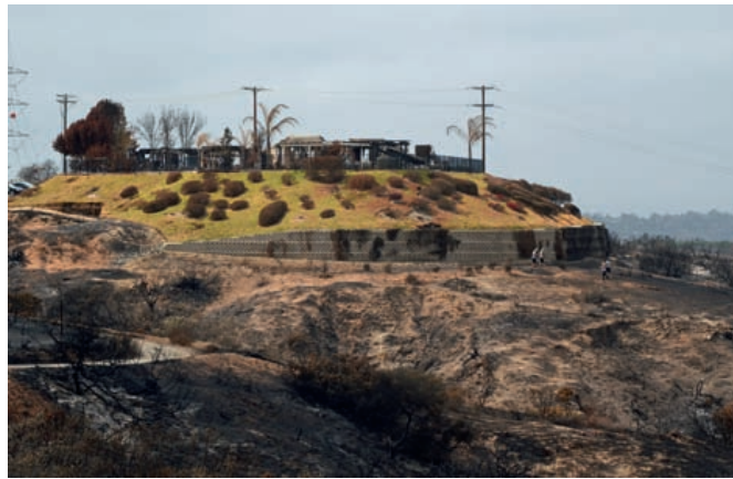
f0015 FIGURE 13.2 Homes burn because they are flammable. Many homes with adequate defensible space still burn in wildland fires because embers land on flammable materials around the home or enter through openings such as attic vents. These two homes burned during the 2014 Poinsettia Fire in Carlsbad, California, despite fire-safe landscaping, a firewall, and thinned wildland vegetation. Focusing exclusively on wildland vegetation clearing ignores the main reasons homes burn: they are flammable. (Photo credit: Richard W. Halsey.)
